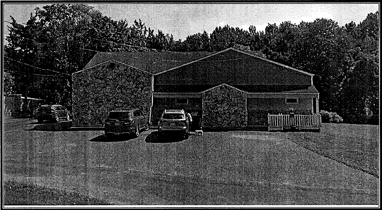
View of existing building
