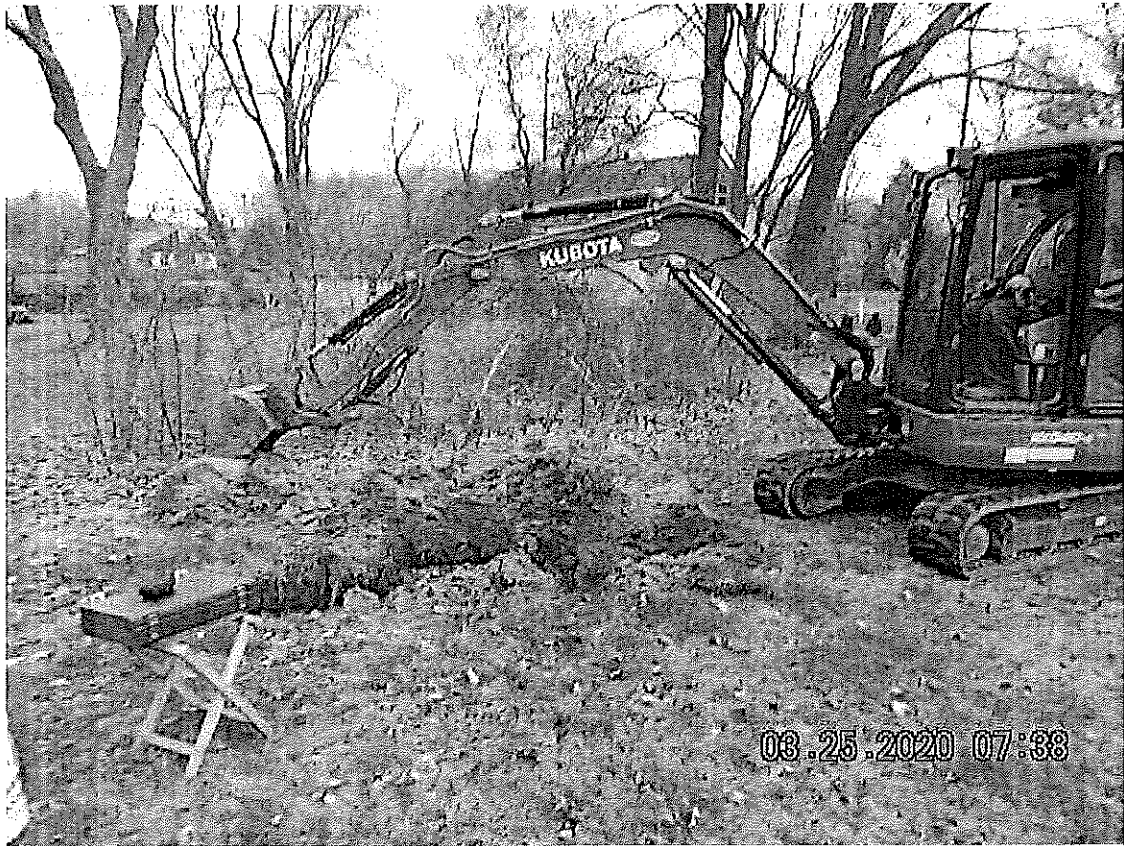
TEST PIT #2 EXCAVATION
