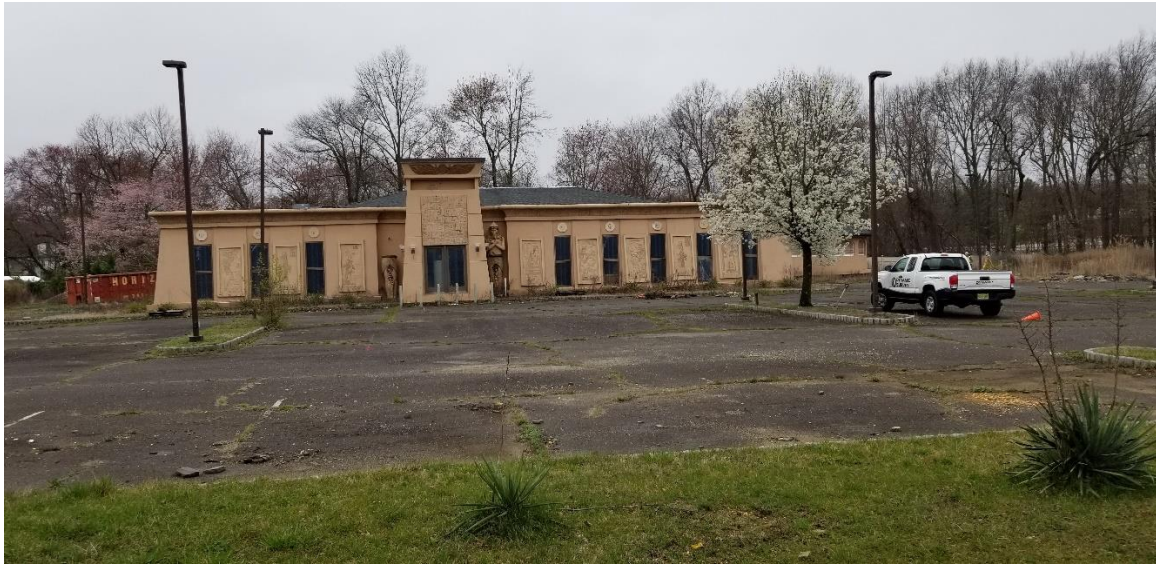
Photo 3: Photo facing west towards the existing vacant restaurant and parking area.
