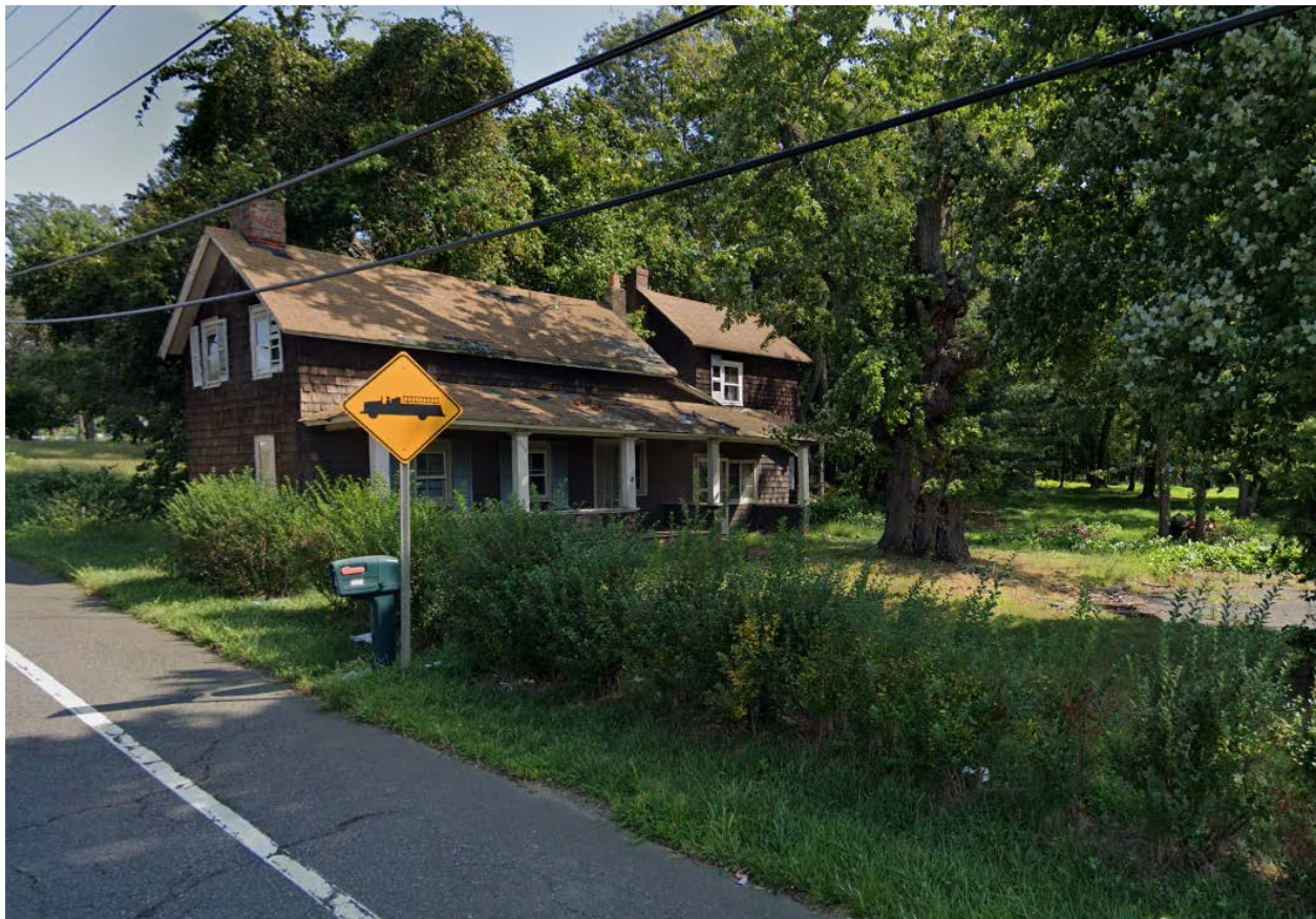
View of existing dwelling (to be demolished)
